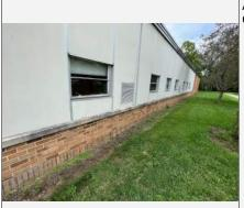
Area for exterior windows / panels in poor condition Cast stone sills needing to be treated for blue-green algae - clean, seal and provide preventative zinc strip
