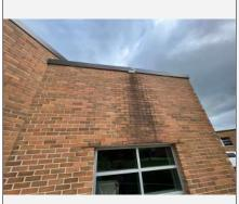
Need to fix drainage scupper to flow away from face of brick
