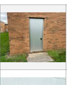
Exterior stoop at exit door needing to be flush with grade
