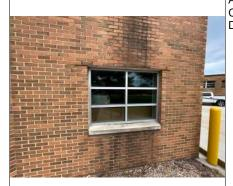
Area of damaged masonry needing to be replaced Cast stone sill needs to be cleaned / sealed Drainage needs to be corrected
