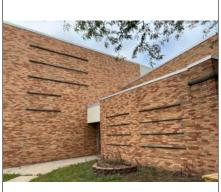
Cast stone details with blue-green algae needing to be treated, cleaned, sealed and a preventative zinc strip added to the top side of the cast stone
