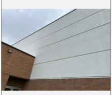
Exterior Insulation Finish System (EIFS) in good condition
