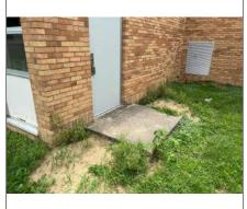
Exterior stoop at exit door needing to be flush with grade
