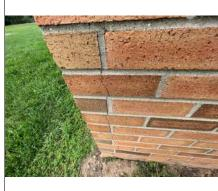
Portion of exterior masonry that is cracking, need to add control joints and replace damaged masonry
